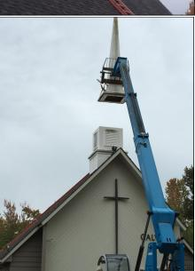
As part of the roof repairs, the steeple was removed due to leakage and mold issues. Many thanks to Mel McCracken for coordinating the project.
